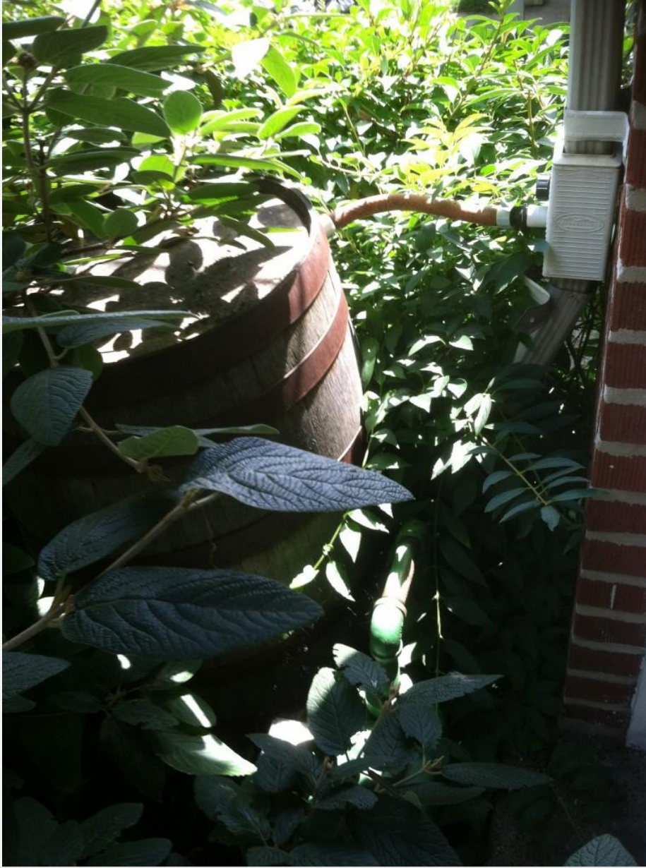
A rain barrel attached to a home drain spout.
